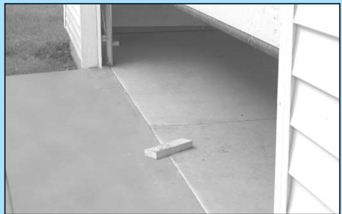
FIG. 6-5 2 x 4 under center of door opening.
