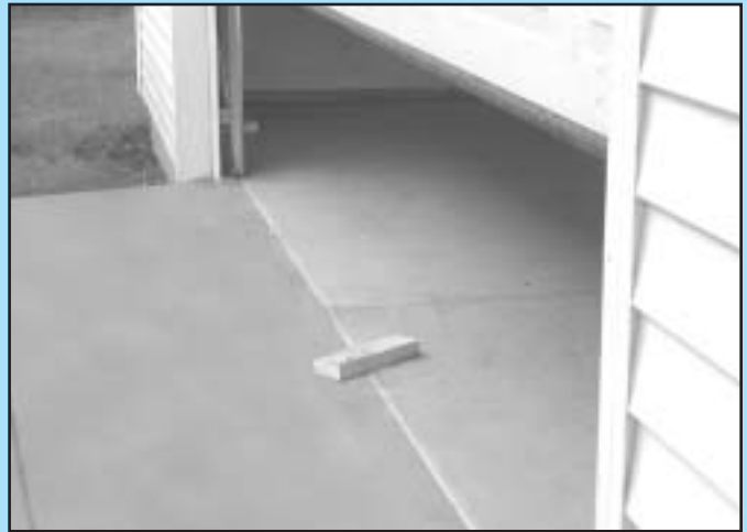
FIG. 7-5 2 x 4 under center of door opening
