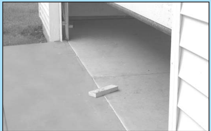
FIG. 6-5 2 x 4 under center of door opening.
