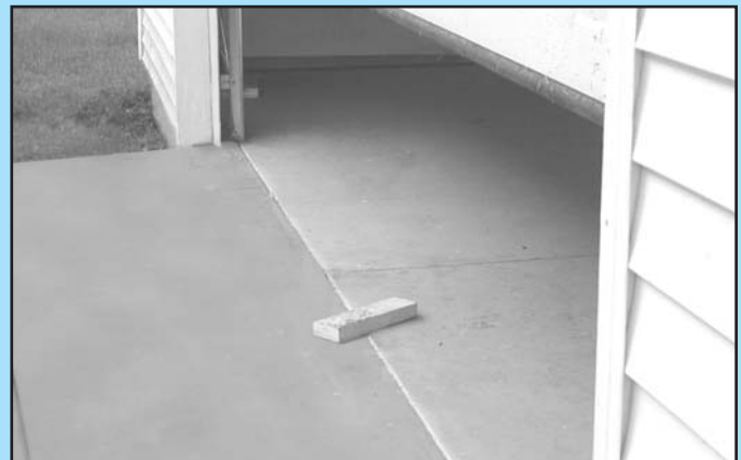
FIG. 6-6 2 x 4 under center of door opening.
