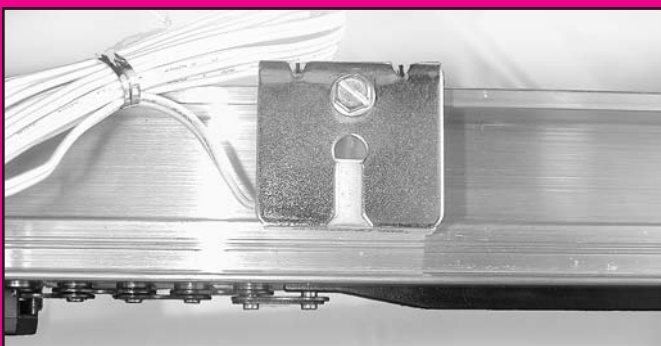
FIG. 7-2 Place "Open" limit switch.
