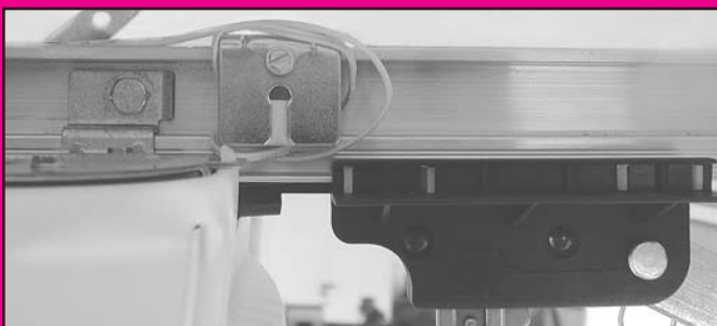
FIG. 7-4 Align "OPEN" limit switch.
