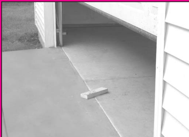
FIG. 7-5 2 x 4 under center of door opening.
