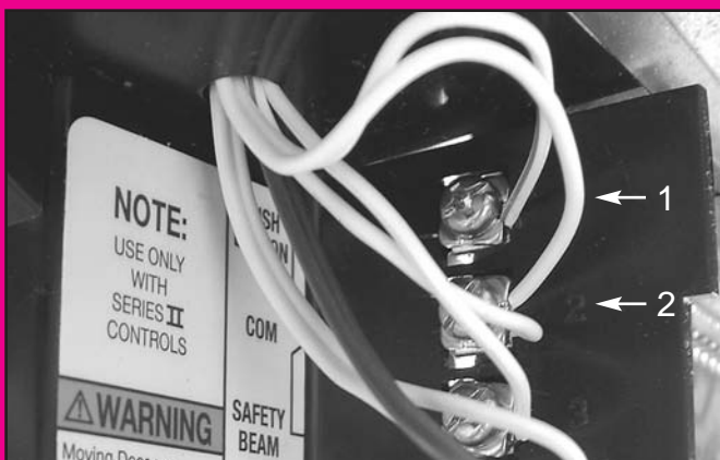
FIG. 5-1 Terminal attachments at power head.
